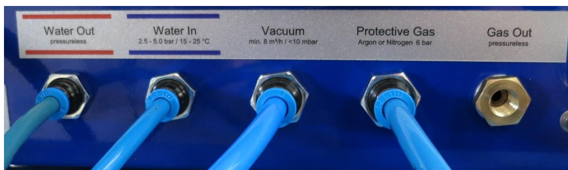
Figure 15: Check of the backside connections
